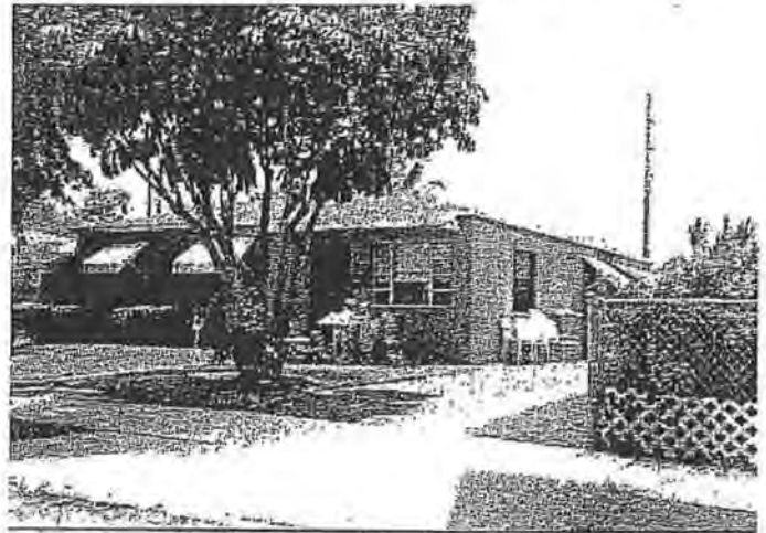
An Existing Quality Home Serves as an Example for Residential Redevelopment Potential
