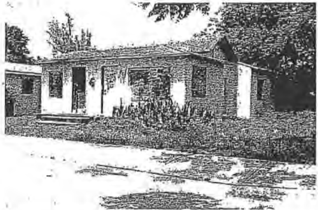
Abandoned Residential Property in the Heart of the Redevelopment Area
